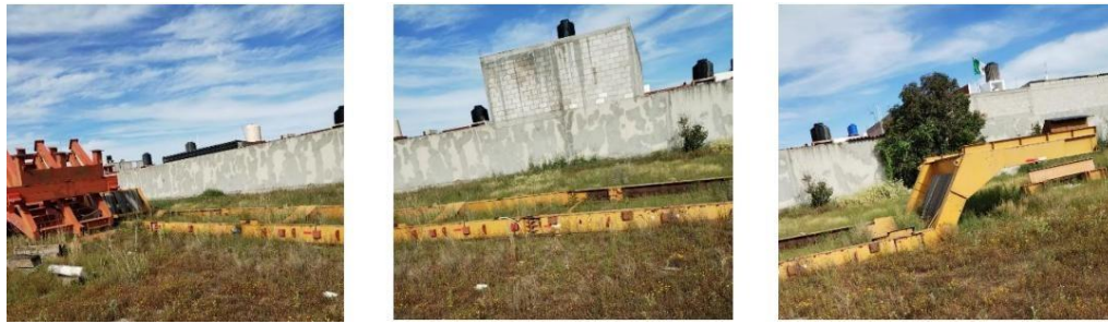
Fig. 2. Current Condition of the Tanker Platform (Own elaboration)
