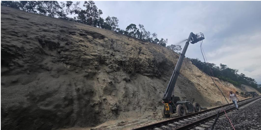
Fig. 2. Shotcrete with prior trimming, Section 7 of the Maya Train. Source: Author's own.
