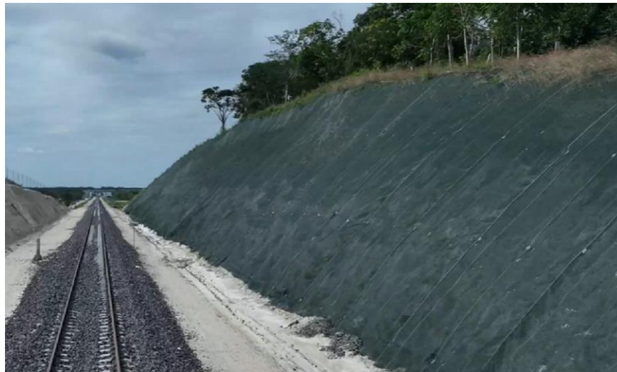
Fig. 1. Geomat and hydroseeding, Section 7 of the Maya Train. Source: Author's own.
