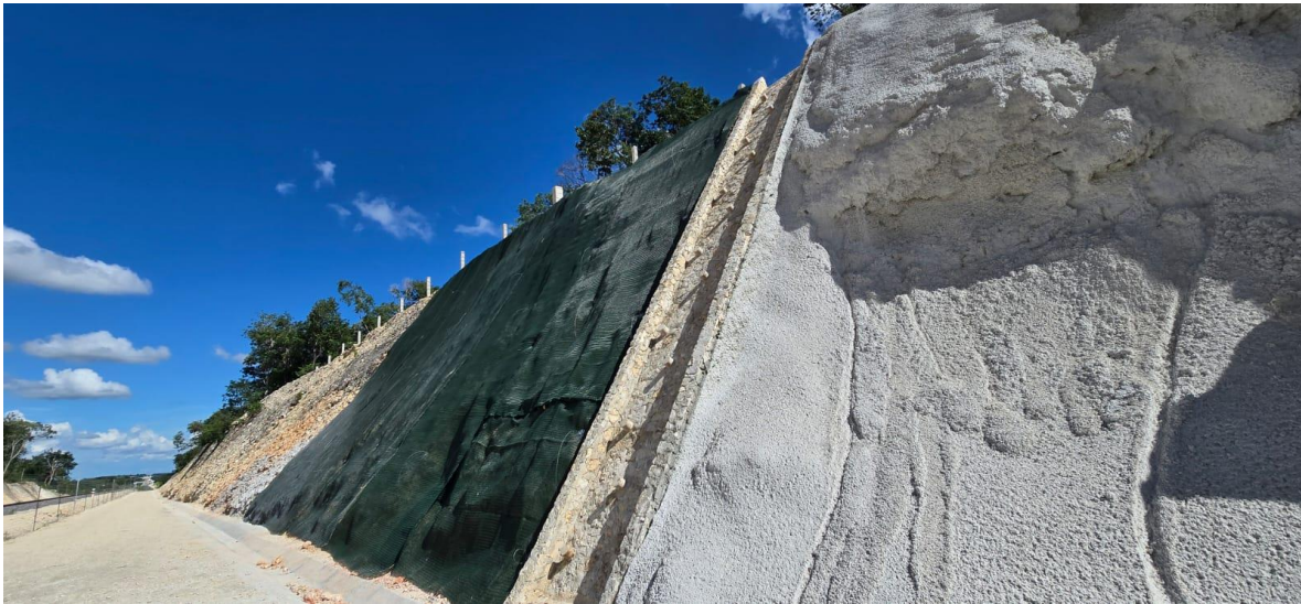
Fig. 4. Integral stabilization with drainage and structural treatment, Section 7 of the Maya Train. Source: Author's own.
