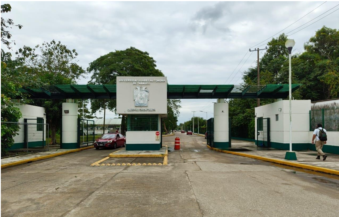
Fig. 1. Single entrance to the Chontalpa Campus.
